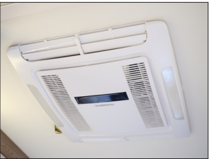
Klimaanlage – Dometic Fresh Jet FJ2600
